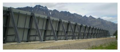
BlastWall is a patented all-fiberglass blast fence with the structural strength to withstand jet takeoff blast and remain invisible to radar and radio transmissions. It is engineered to deflect a blast of 160 km/h at a safety factor of 1.5:1, yet has sufficient frangibility to collapse upon impact without major damage to aircraft or BlastWall.
