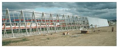
BlastWall has been tested extensively by NAV Canada for non-interference performance during ground based and in-flight electronic signal emissions. It has been engineered to meet or exceed NAV Canada airside installation requirements and has been approved for installation in airports across Canada.
