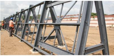
All the components of BlastWall, including the nuts and bolts, are made from pultruded or molded fiberglass to create a lightweight and durable structure with no metal parts. Pigment and UV stabilizers are incorporated into the fiberglass resin to make it corrosion-resistant and maintenance free.
